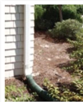
*Left: example of a downspout that contributes to stormwater pollution; Right: an example of a redirected downspout that infiltrates and prevents stormwater runoff.*
