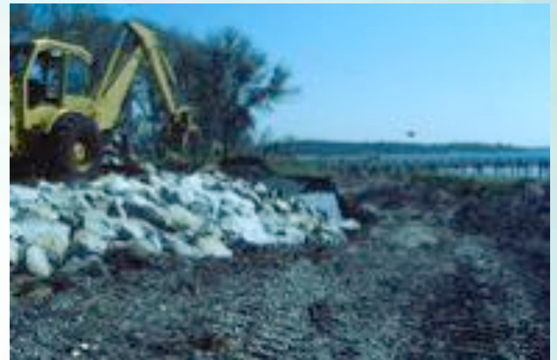
Bogue Sound Revetment During Construction - 5/98
