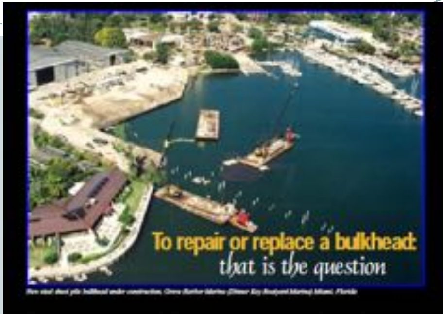
Replacement steel sheet pile bulkhead under construction, Bahia Acahuacal Yachting Center, Ft. Lauderdale, Florida
