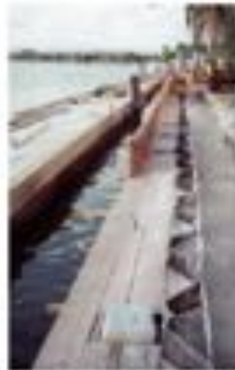
Replacement steel sheet pile bulkhead under construction, Bahia Acahuacal Yachting Center, Ft. Lauderdale, Florida
